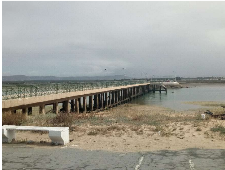
Figure 2.2. Sampling station 1 – Bridge of Faro Beach.
